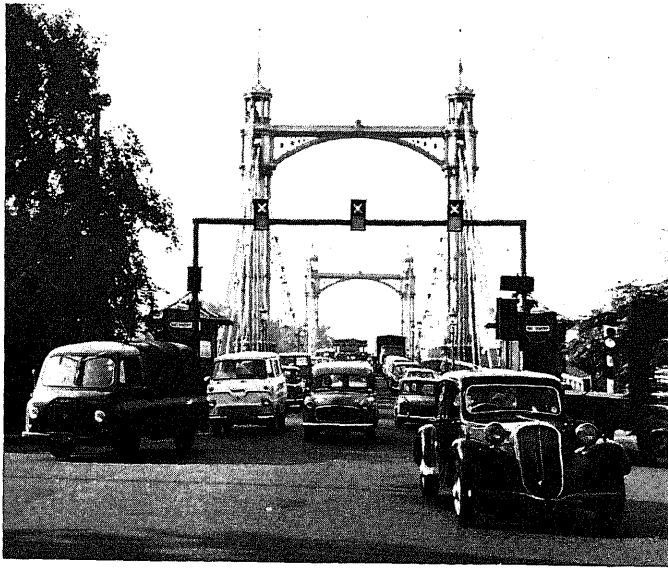
One-way tidal flow on Albert Bridge: morning flow into Central London
