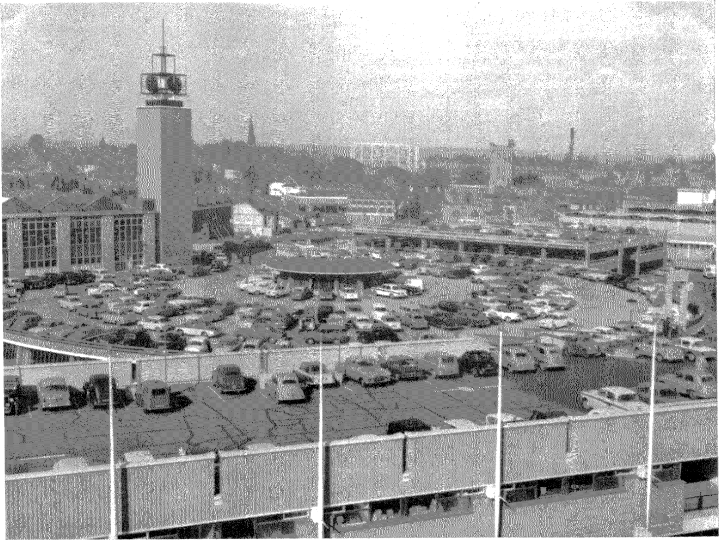
System of linked roof-top car parks at Coventry
