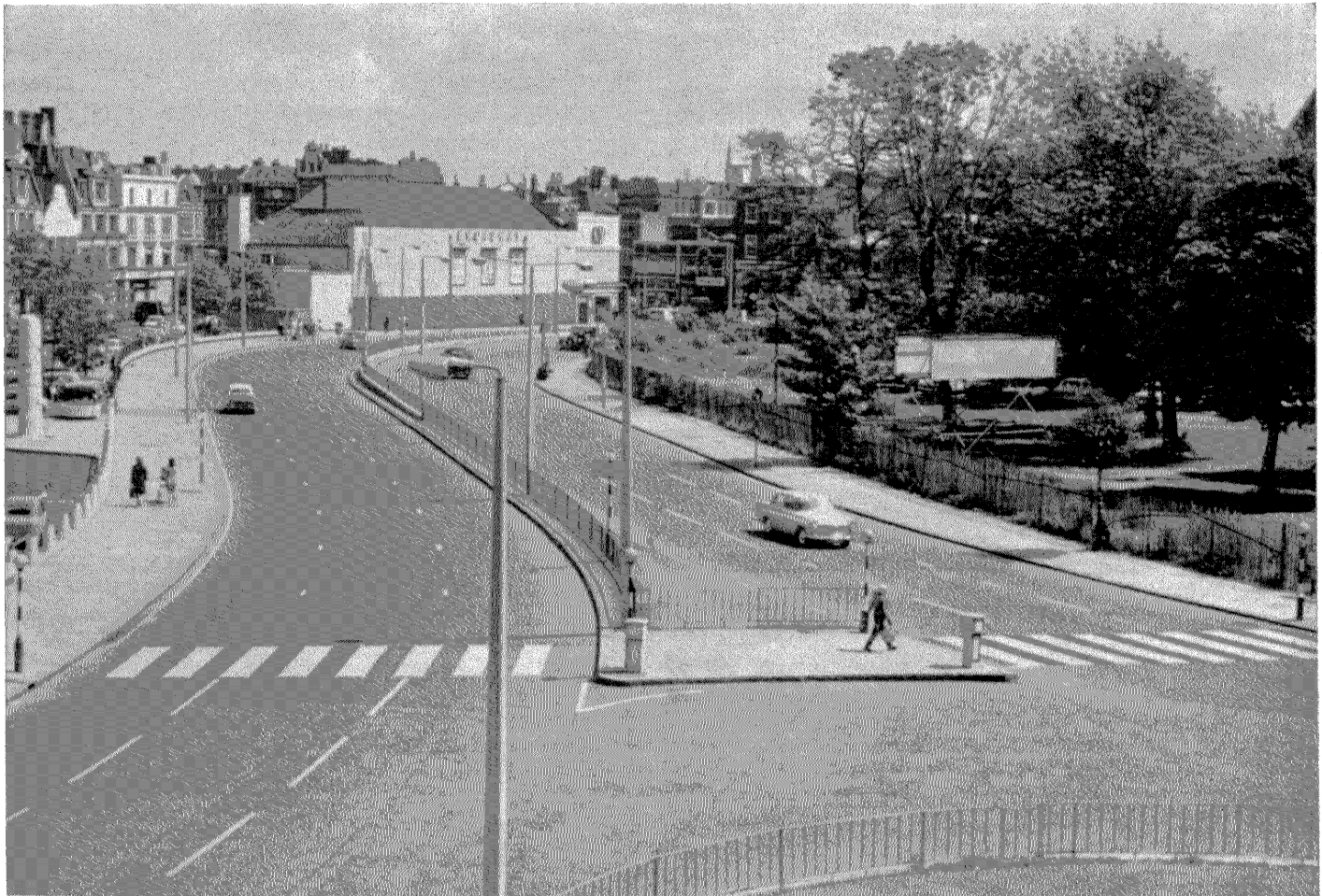
Fences should not restrict visibility at bends or junctions, or conceal pedestrians at crossing places
