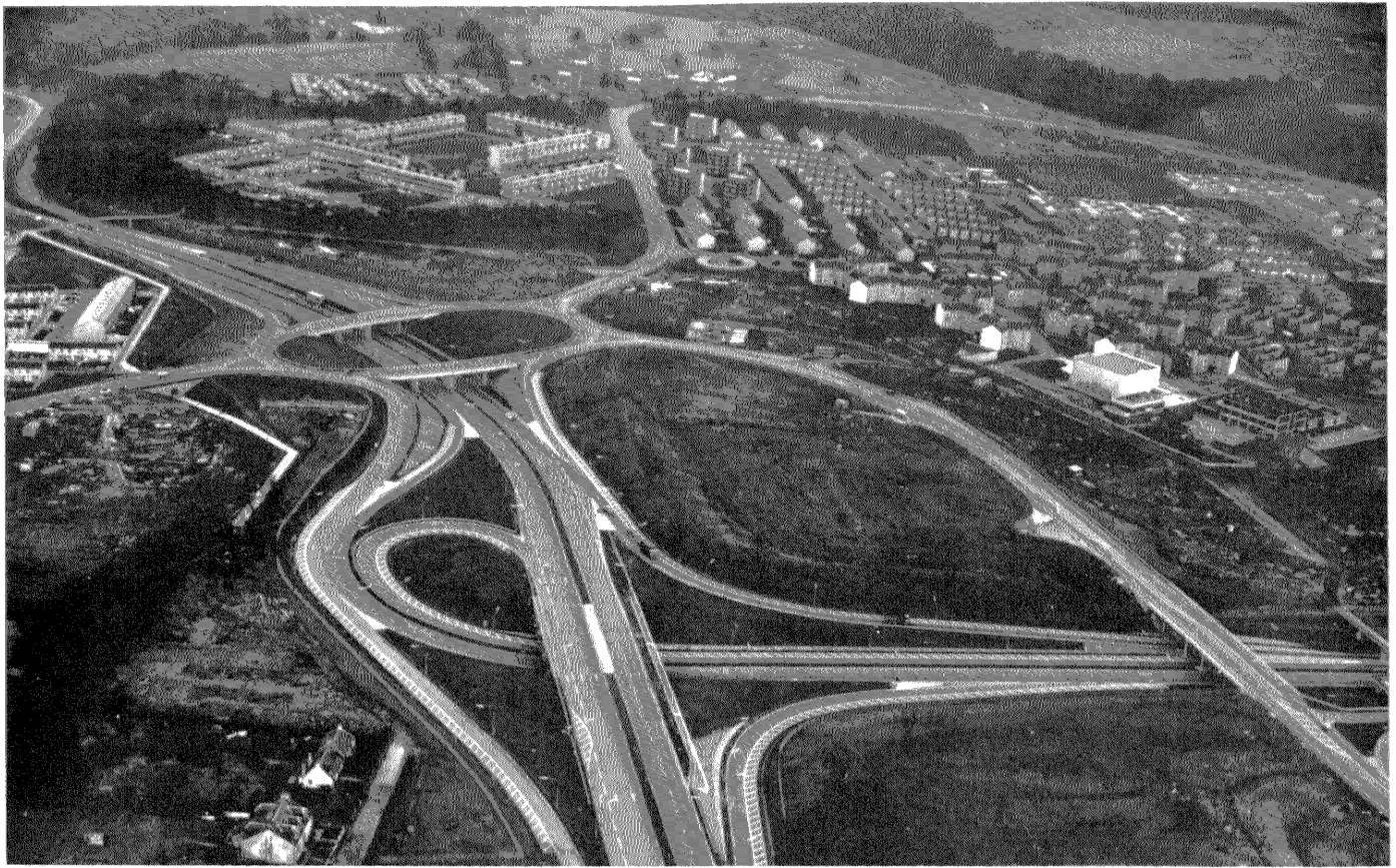
Distributor roads and interchanges at Cumbernauld ( reproduced by courtesy of the Cumbernauld Development Corporation )
