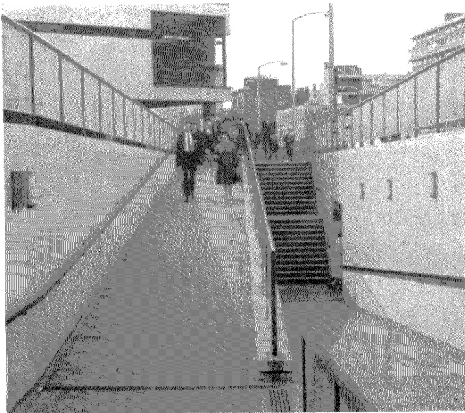
Subway with ramped approaches as well as steps
