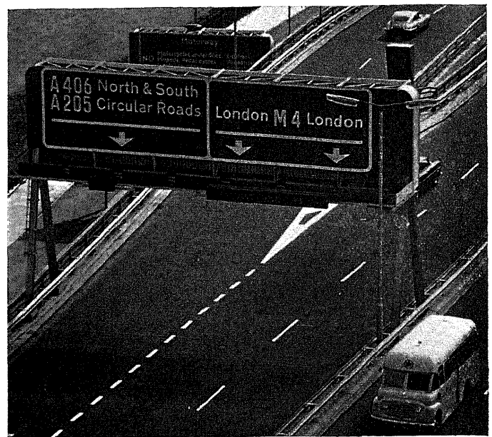
Gantry sign at exit slip road from Motorway M.4
