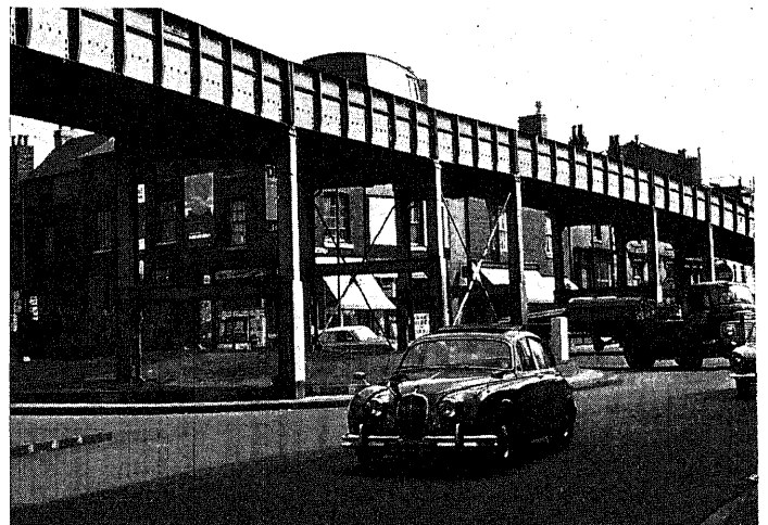
Temporary flyover at a congested junction in Birmingham
