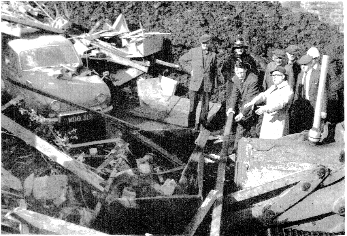
1.22 Photograph taken at approximately 11.15 a.m. on 21st October 1966 showing relatively 'dry' nature of rubbish with no indication of free water on the road surface.
